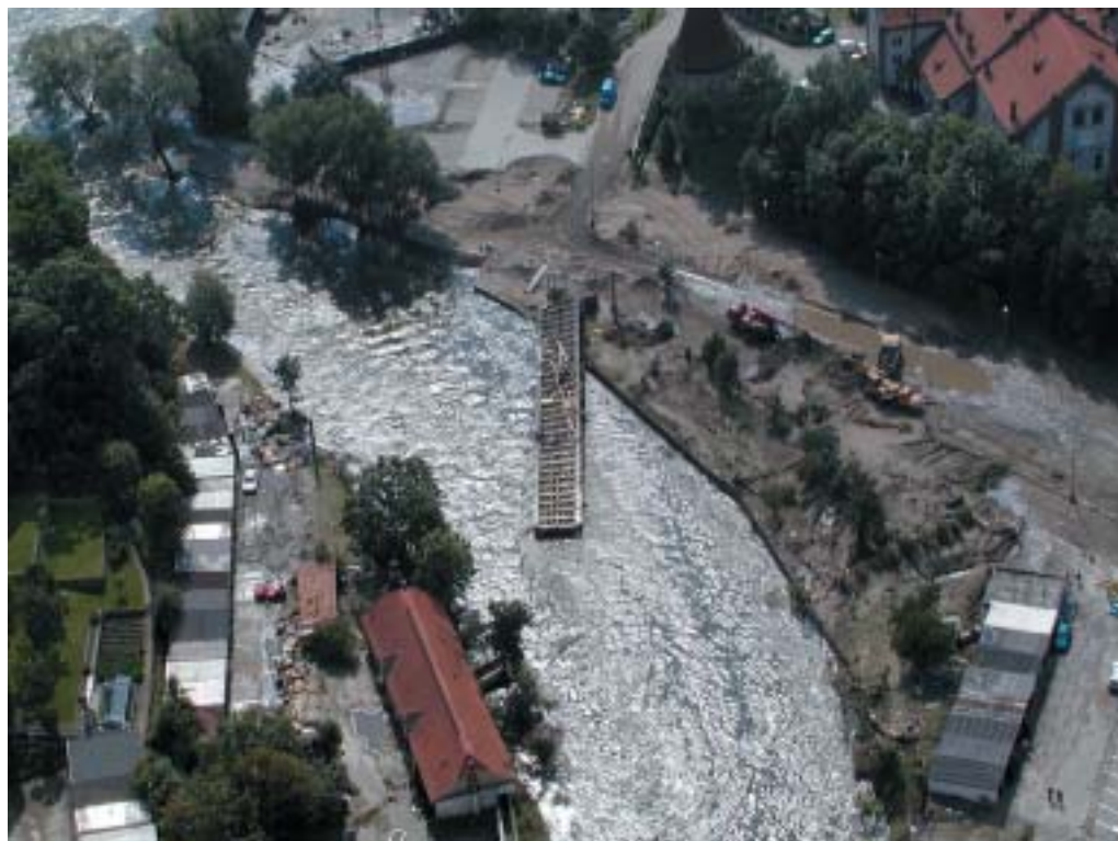
Flood Damage along Vltava River, Czech Republic, August 2002
